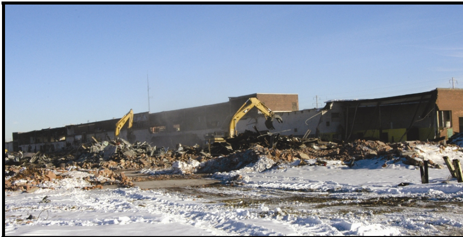
Detroit Artillery Armory Demolition Eight Mile Rd. Oak Park, MI
