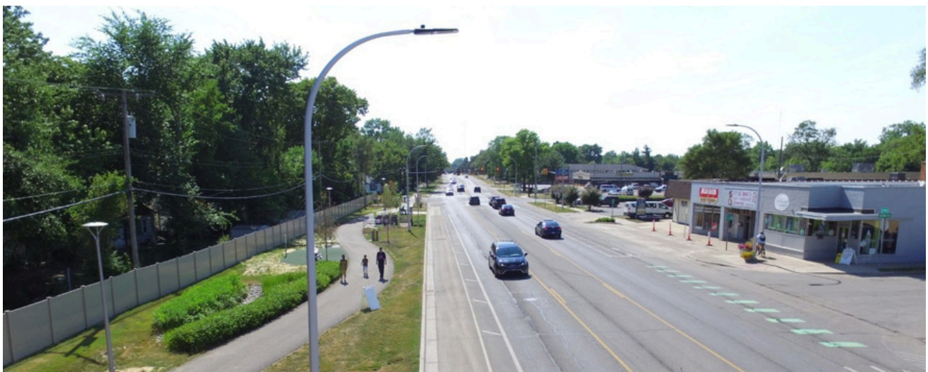
Street view: Nine Mile Westbound
