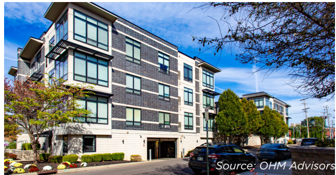
Source: OHM Advisors Podium parking under residential flats with controlled access and overhead door. This parking also extends below an adjacent amenity deck (courtyard).
