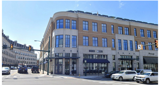
Tall first floors make opportunities for versatile high-quality commercial space. Upper floor is stepped back to reduce apparent building height. Source: Google Earth
