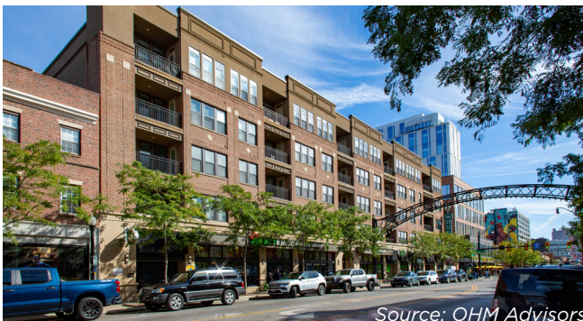
First floor commercial should provide storefront windows for the display of goods and services. Source: OHM Advisors
