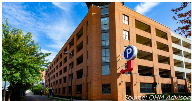
Source: OHM Advisors 6-level parking structure has borrows materials and opening proportions from adjacent office mixed-use buildings.
