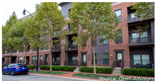
Source: OHM Advisors Flats with common entry for upper floors, and individual unit entries for first floor adds activity to the street.
