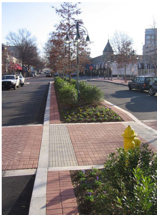
Landscaped median islands can bring the aesthetic treatments into the roadway, while providing a safe and comfortable place for pedestrians to cross the street. Source: NACTO
