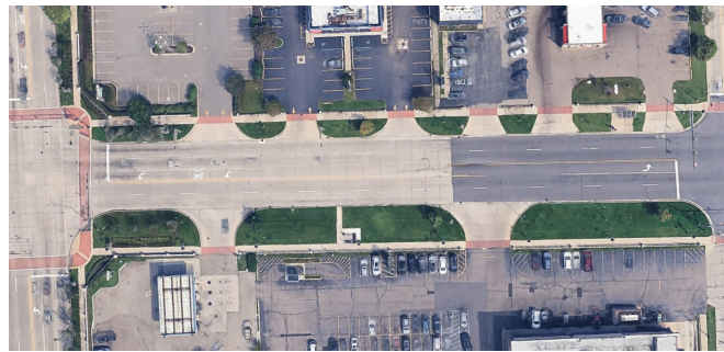
The driveway spacing along the north side of Nine Mile Road, east of Coolidge Highway contributes to the high density of crashes and negatively affects traffic operations at the intersection. Source: Google Earth.
