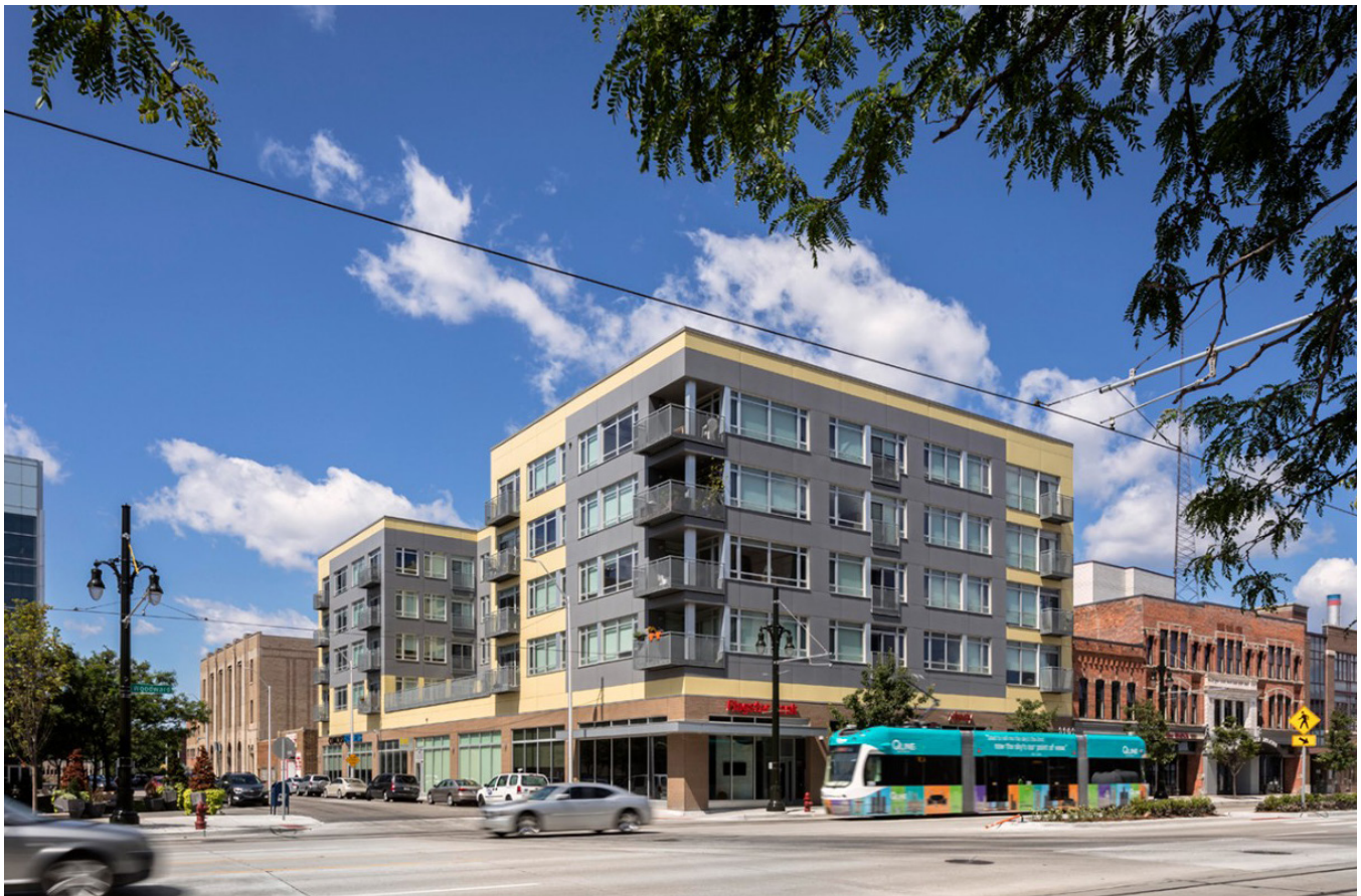
Woodward Garden Apartments in Detroit, MI was financed with the assistance CDBG loan-guarantee program Source: McIntosh Poris Architects
