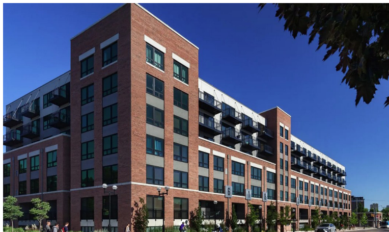
618 South Main in Ann Arbor offers a 150 units and full amenities. The project was awarded $3 million in Community Revitalization Program performance-based loan and $3 million in Brownfield TIF funding Source: Clayco Farmington
